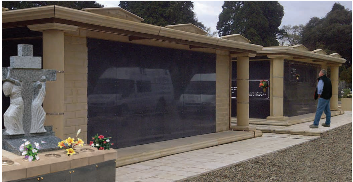
A second phase work in progress installation of welters® Majestic Mausoleum incorporating a mix of front and side charging interment options with granite tablets for inscriptions and an attractive communal planter arrangement.
