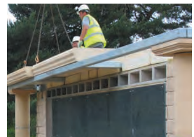
Specially design roof panel section installation
