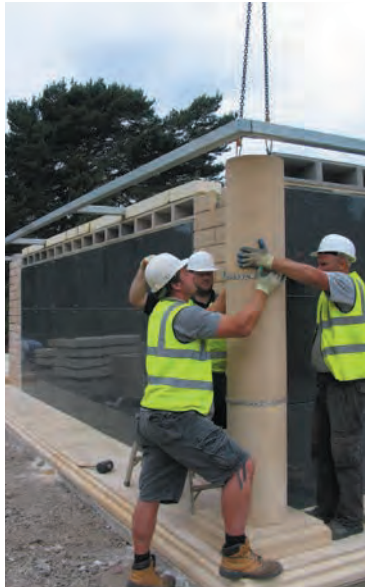
Circular column installation
