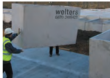
Burial Chamber Installation in saturated land
