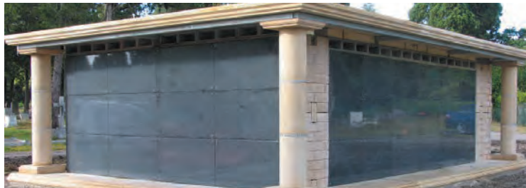
welters® Majestic Community Mausolea - work in progress
