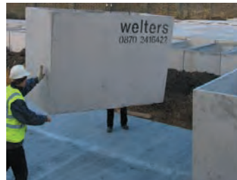
Burial Chamber Installation in saturated land
