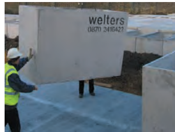
Burial Chamber Installation in saturated land
