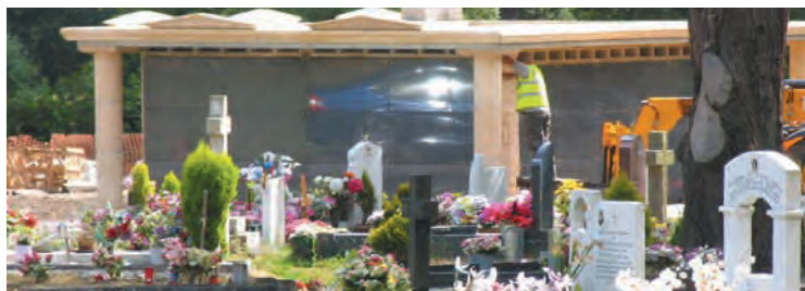
welters® Majestic Community Mausolea - work in progress
