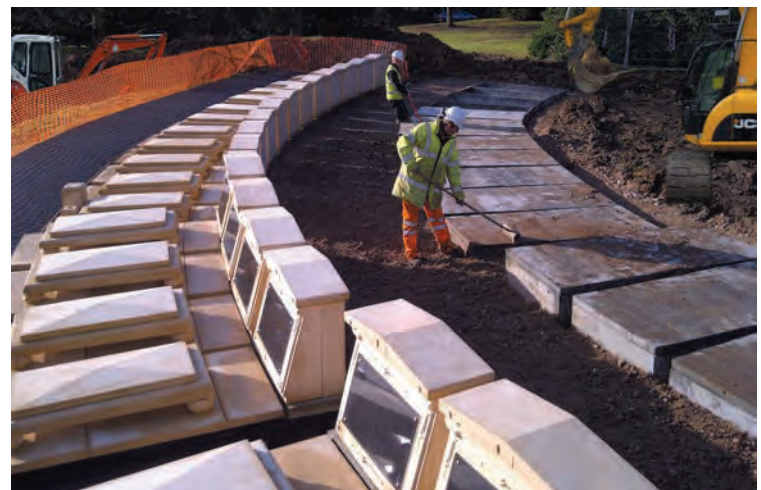
Double Interment Concentric Chamber installation above existing graves - second phase installation under construction. Virtual representation shows the finished second phase development with a decorative octagonal centre feature. The below ground interment provision can be seen from this vantage point.
