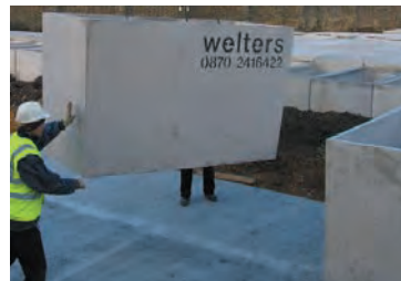
Burial Chamber Installation in saturated land
